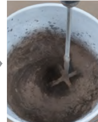
Ready for Grouting
